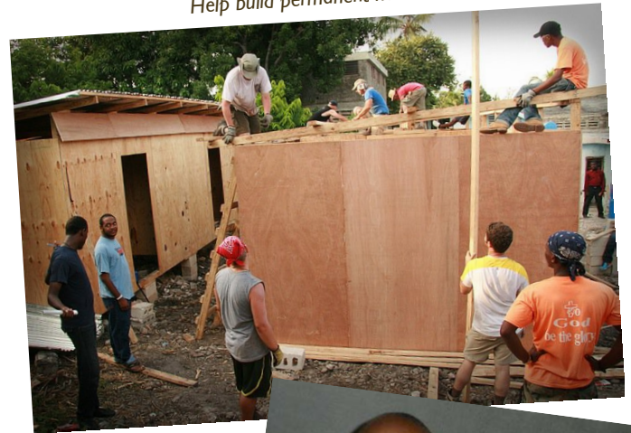
Help build permanent homes
