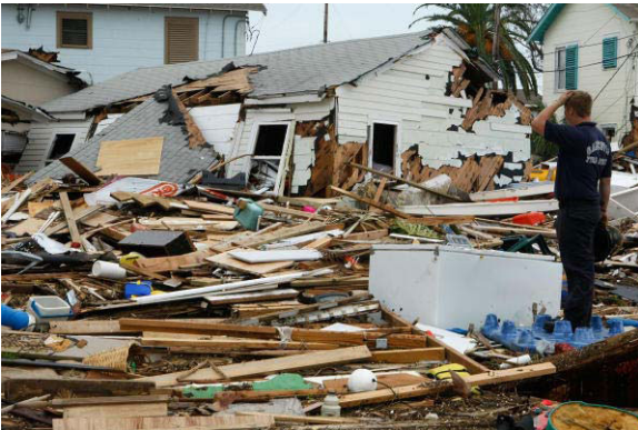
Surveying the damage post-Ike.
