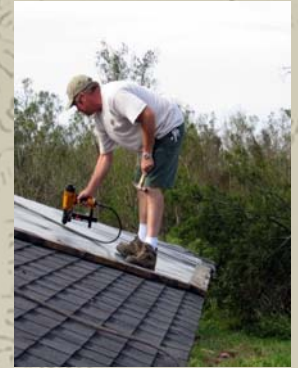
A volunteer repairs a roof.
